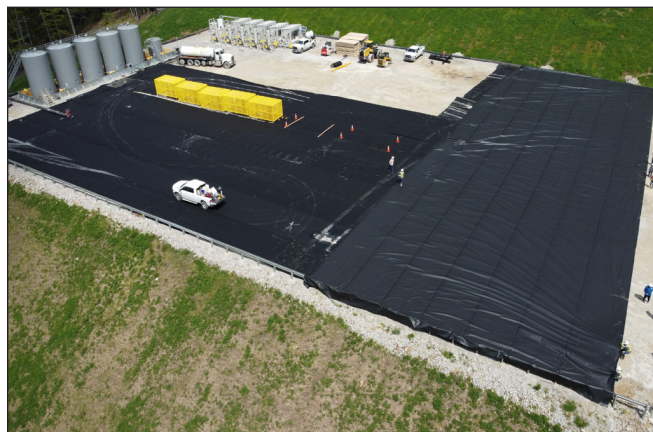
Rig Pad Liner
