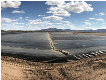
Full site deployment of the Dura-Skrim® RPP panels and ballast tubes
