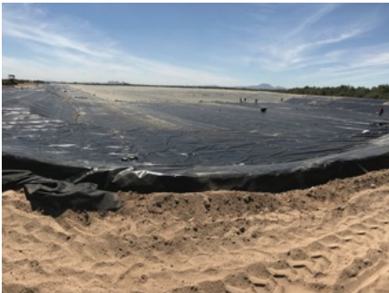
Anchor trench of pond lined with Dura-Skrim® RPP liner to prepare for anchoring the perimeter
