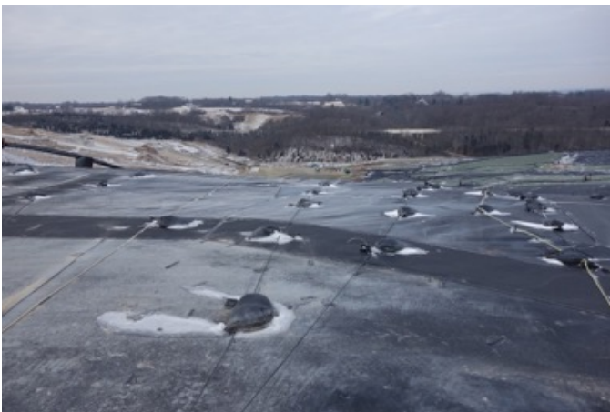
Area with Absolute Barrier® X60 geomembrane cap installed
