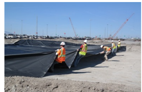
Panel of Y30BAC being opened and installed into place
