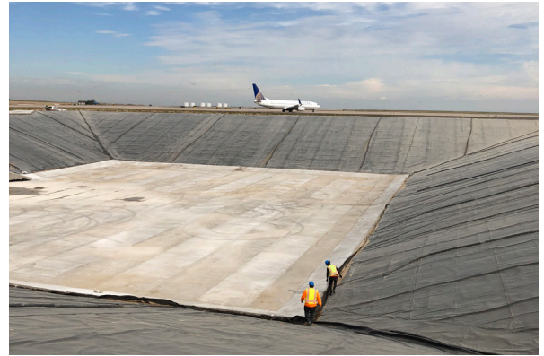
Factory-assembled panel of Absolute Barrier® Y30BAC
