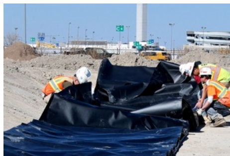
Packaged panel being opened and unrolled into place
