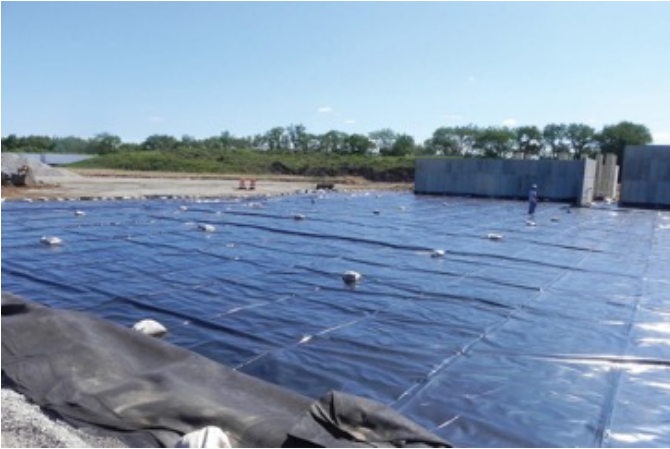
Large prefabricated panels of Absolute Barrier® 25-mil evoh enhanced geomembrane, designed to meet the site's requirements
