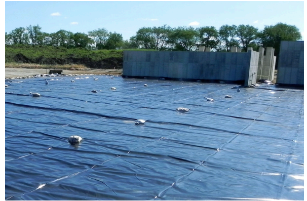
Installation of the secondary containment system utilizing Absolute Barrier®
