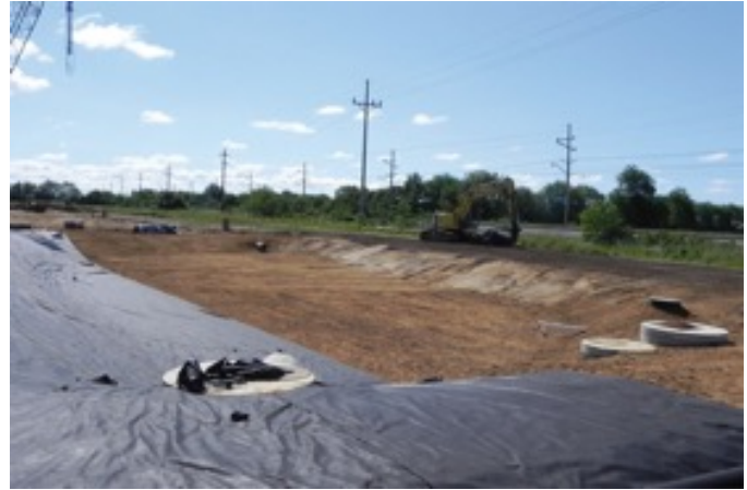
Installation of the secondary containment system
